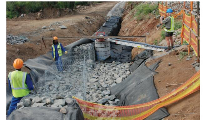
The sump area of a cut-off trench that collects the sub-surface seepage water.
